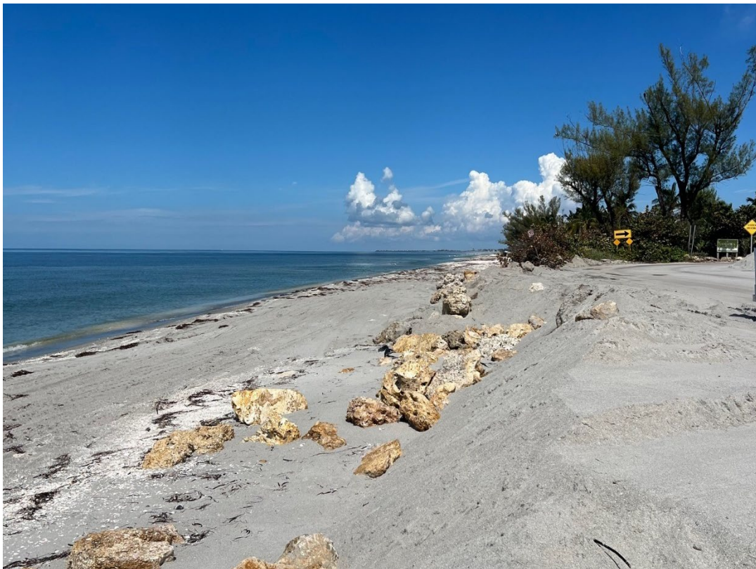
Figure 9. Erosion near Jensen's Curve from Hurricane Helene.
