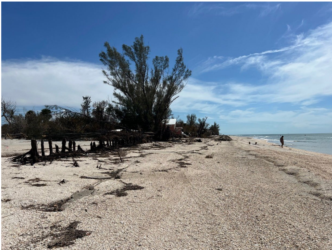
Figure 14. Erosion of beach south of Alison Hagerup Park from Hurricane Milton.
