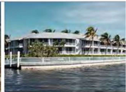
FENEX flood-proof glass walls, Ft. Lauderdale
