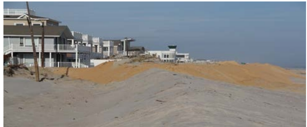
Sand dune protected these homes from Hurricane Sandy. To the north where there was no dune, homes were destroyed. Note new sand already added to replenish the dune to protect against the next storm. (Photo courtesy Emma Lee/NewsWorks)
