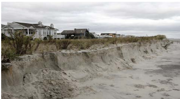
The dune saved these homes in Stone Harbor, NJ. (Photo courtesy Elizabeth Robertson/The Philadelphia Inquirer)
