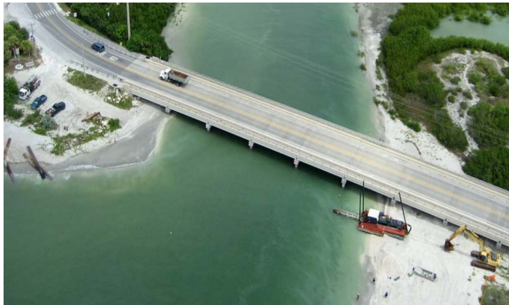
Blind Pass in 2009 after dredging.
