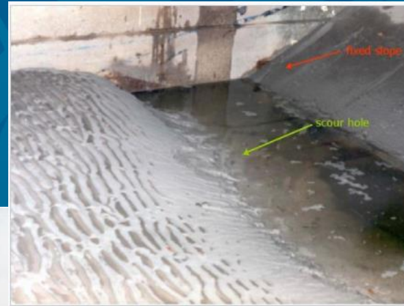
Figure 4 Scour in front of a revetment; Delta Flume test
